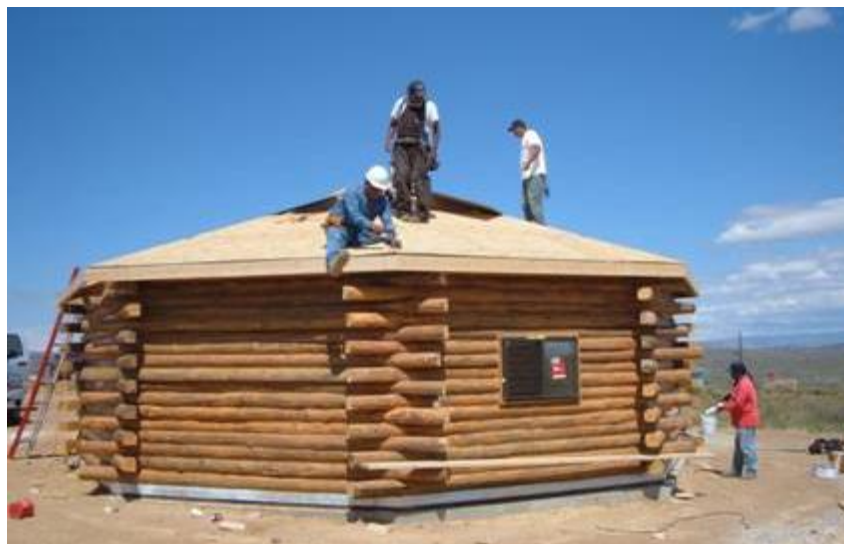
A Navajo traditional home, or hogan, being built with a Forest Service Collaborative Forest Restoration Program grant.
